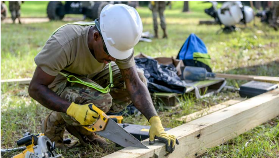
U.S. Army National Guard Soldiers with the 1223rd Vertical Engineering Company, South Carolina National Guard, built an air assault obstacle course at McCrady Training Center in Eastover, South Carolina, June 10, 2021. The engineers built the course as part of their two-week annual training in order to practice their skills of building structures and maintaining their mission readiness as a unit. The course is intended for future training events at McCrady. (U.S. Army National Guard Photo by Spc. Josiah Lining, 108th Public Affairs Detachment)
